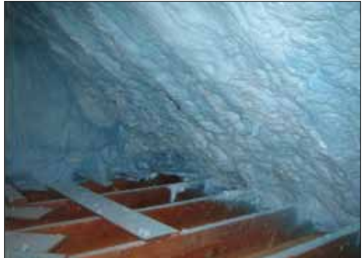
Figure 7 Polyurethane foam used in the rafters
