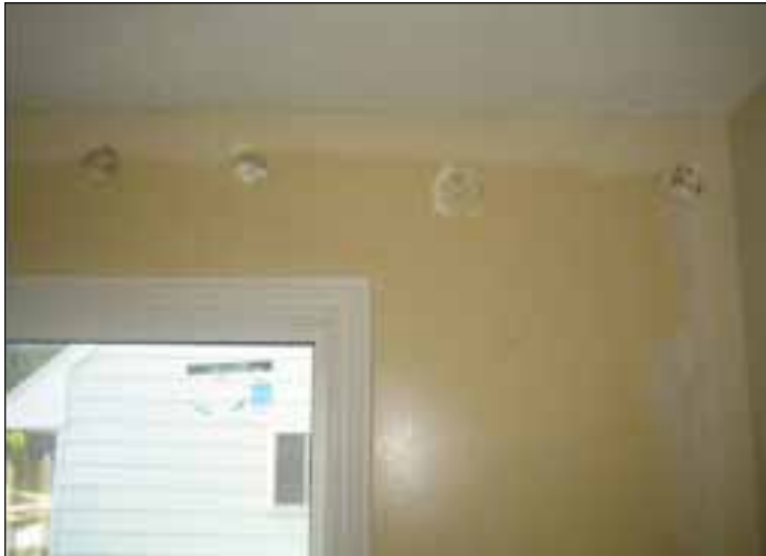
Figure 6 Access holes used to apply polyurethane foam
